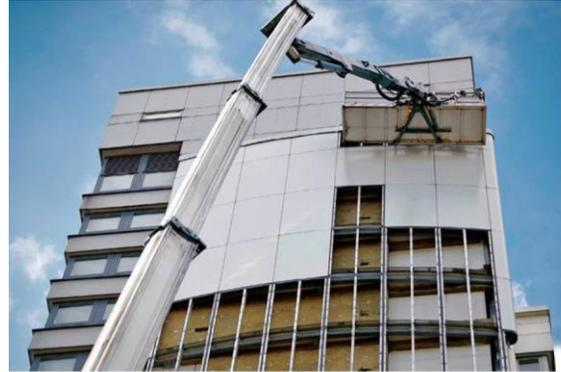
Construction workers remove combustible cladding from an apartment building in London in 2017. The work is costly and complicated, like “trying to peel a huge potato...and put a new skin on it,” according to one expert. Photograph: Getty Images
